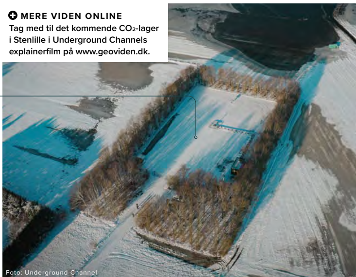
Foto: Underground Channel
